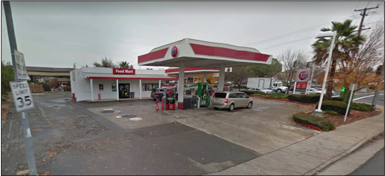
Figure 2: Existing Sierra Food & Gas Site – View from Sunrise Avenue
