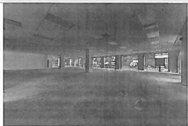
TYPICAL UNIT INTERIOR
