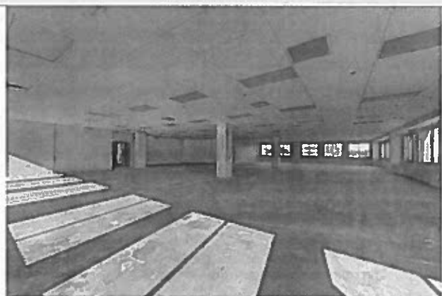
TYPICAL UNIT INTERIOR
