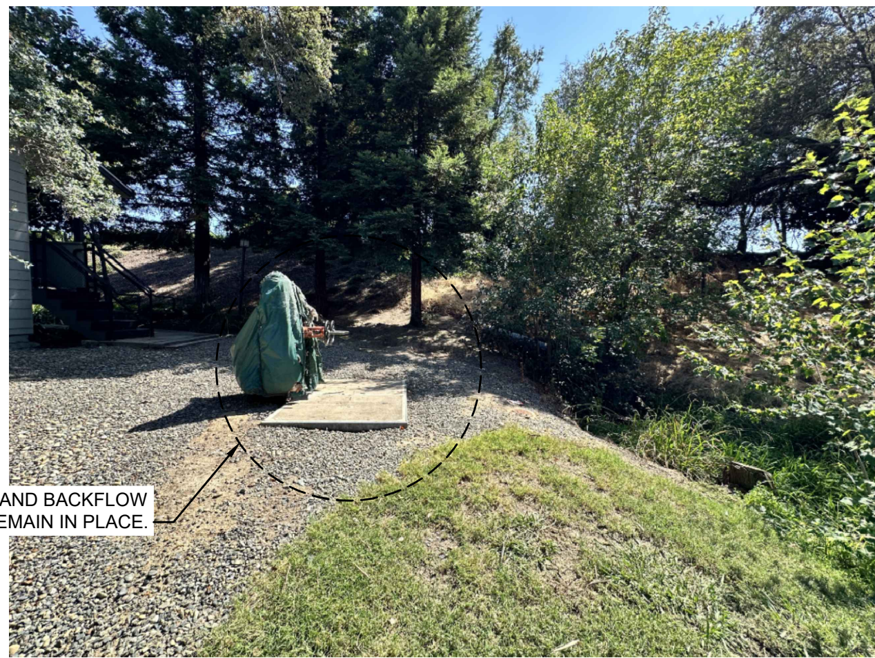
SITE PICTURE: EX METER & BACKFLOW TO REMAIN
