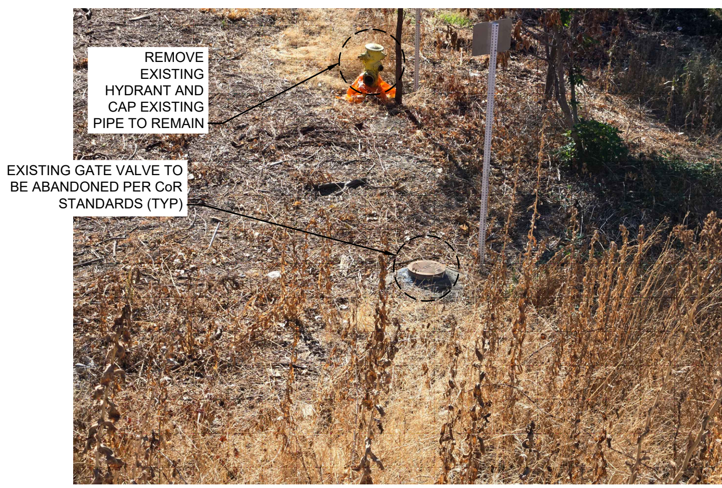
SITE PICTURE: EXISTING BLOWOFF TO BE ABANDONED
