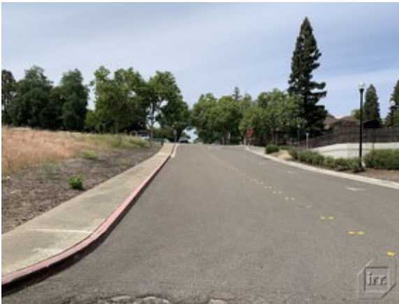
Looking northwest along Taylor Road
