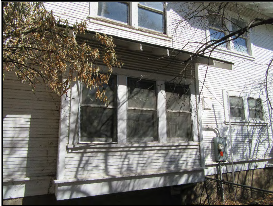
Figure 11. Boxed oriel windows with shed roof on the southern elevation (view toward north), September 26, 2019.
