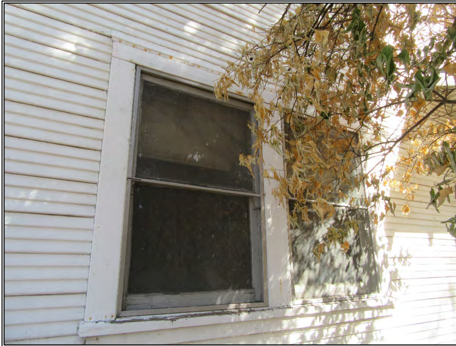
Figure 13. Wood-framed, single-hung windows, southern elevation (view toward north), September 26, 2019.
