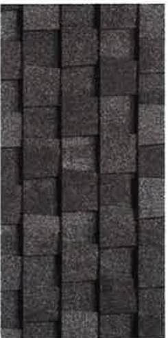
Asphalt Shingle Roof
