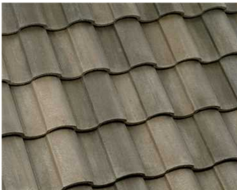
Roof: Eagle - 3687 Brown Gray Range
