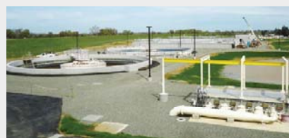
Upgrade and expansion of the existing 1 MGD wastewater plant to a 5 MGD Title 22
