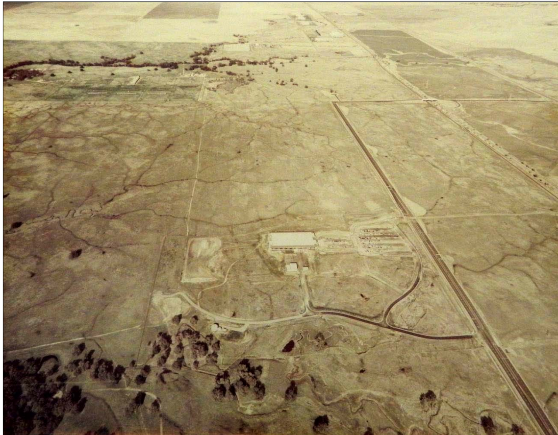
Hewlett-Packard Roseville Campus Initial Construction, 1981
