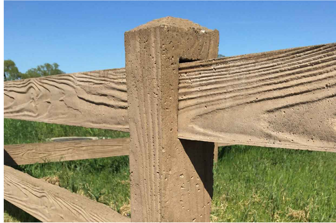
PRECAST TWO-RAIL FENCING: COLOR: 'EARTHTONE BROWN' OR EQUAL MANUF. BY DYNAMIC PRECAST, PHOENIX PRECAST, ARTISAN PRECAST, OR EQUAL INTENT: NATURALISTIC COLOR, FENCING TO VISUALLY RECEDE.
