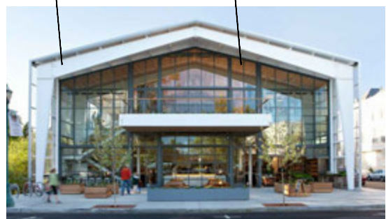
Peaked Main Entry Full Height Glazing
