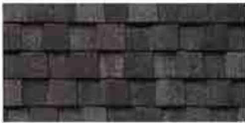
Asphalt Shingle Roof
