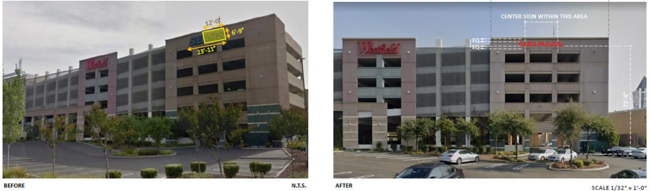
Figure 5: Parking Garage Sign (Before and After)
