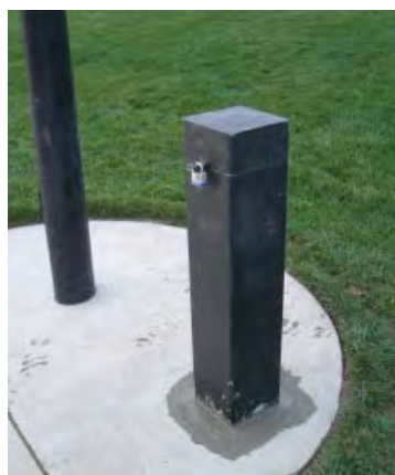
Monitoring well containment box
