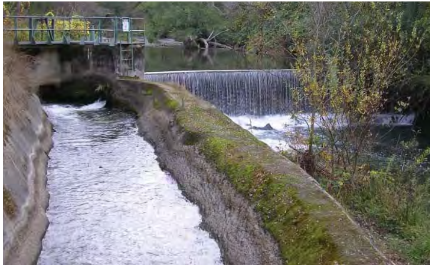
Auburn Ravine Diversion
