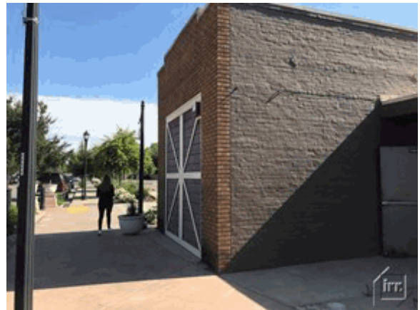
Building exterior (original structure)
