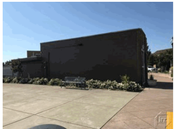
Building exterior facing north
