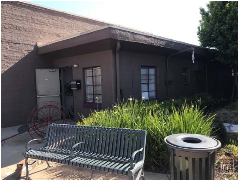
Roseville Fire Station 400 Lincoln St. Roseville, California
