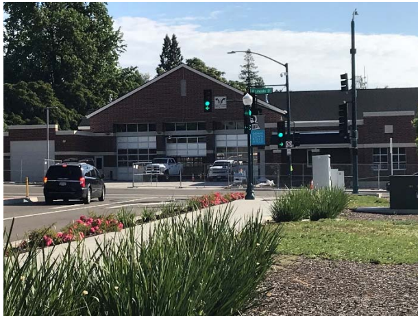
New fire station (80 Lincoln Street)
