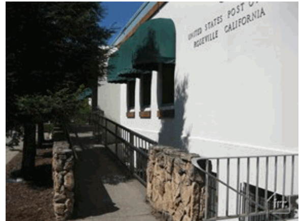
Ramp to main entrance
