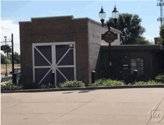
Building exterior facing west (front)
