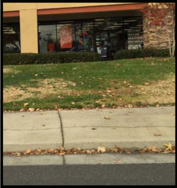
Heavy evidence of runoff
