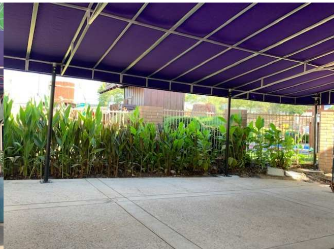
Figure 3. Inside View of Patio
