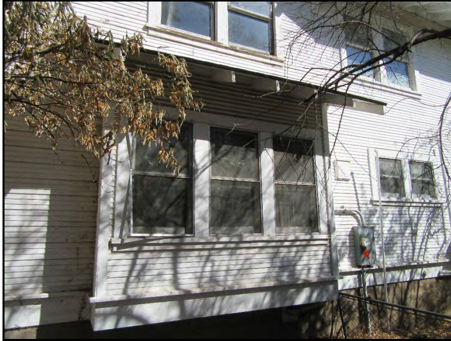
Boxed oriel windows with shed roof building, southern elevation (view toward north).
