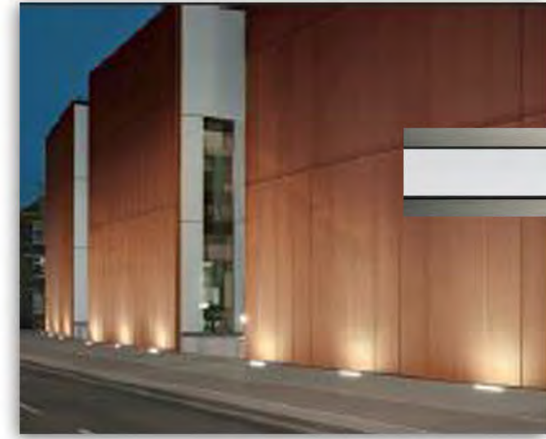
c.) in ground led luminaire
