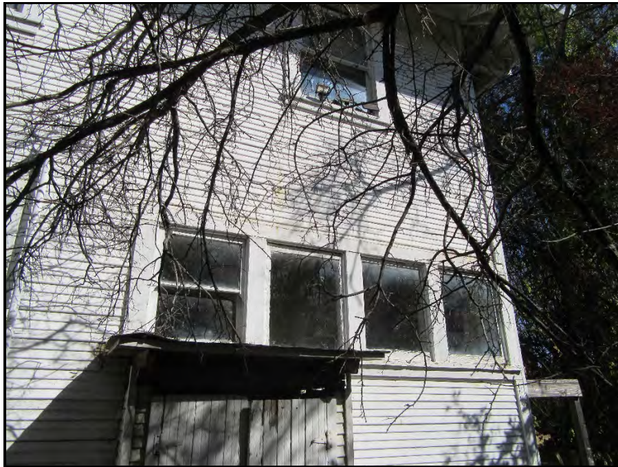
Wood framed, fixed and single hung windows, southern elevation (view toward north).
