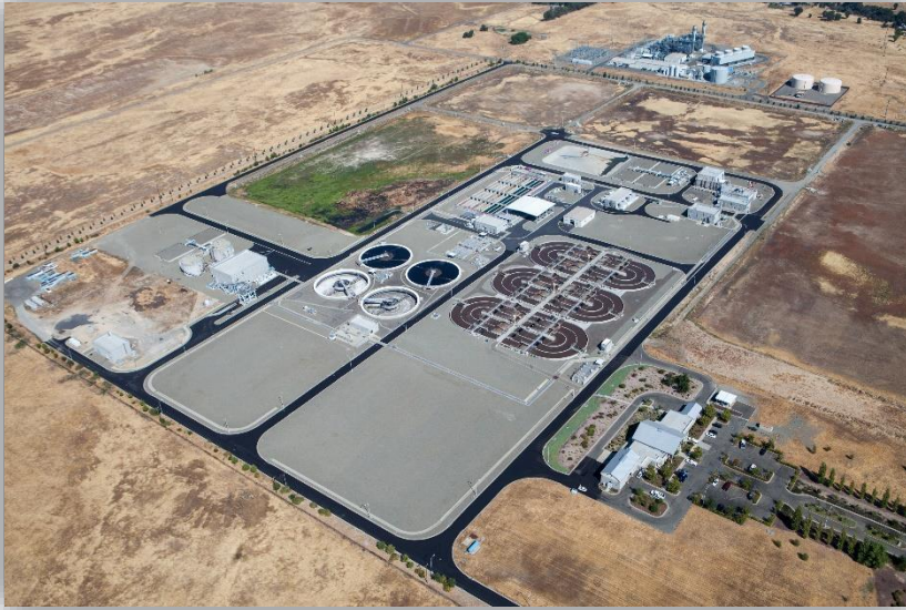
Pleasant Grove WWTP
