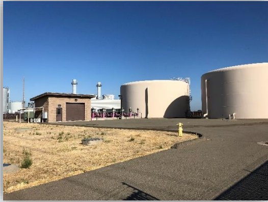
West Roseville Pump Station
