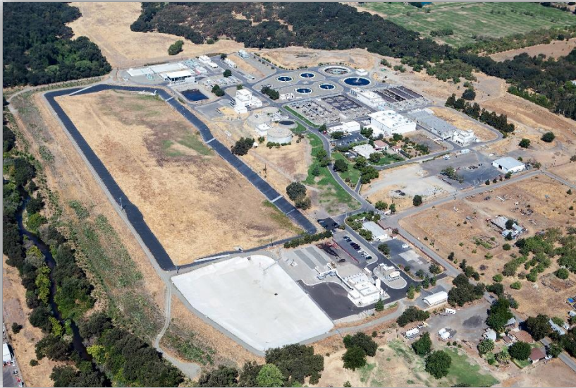
Dry Creek WWTP
