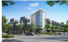
3rd & S Apartments, Sacramento CA
