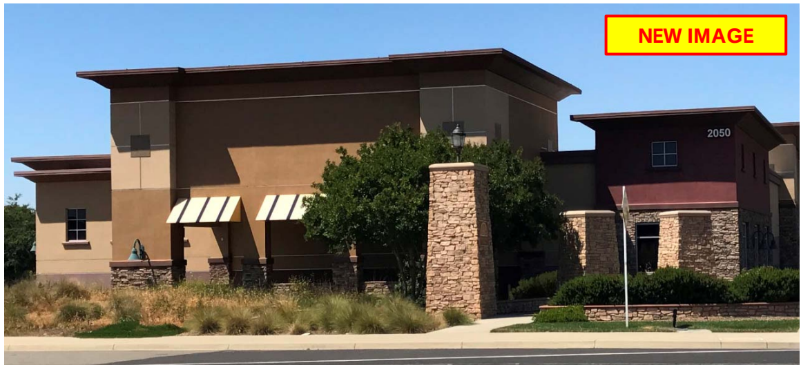
Typical Commercial Roadway
