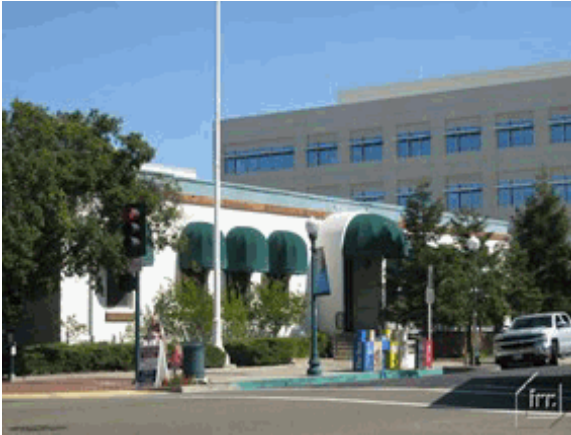
Building exterior facing southeast – main entrance
