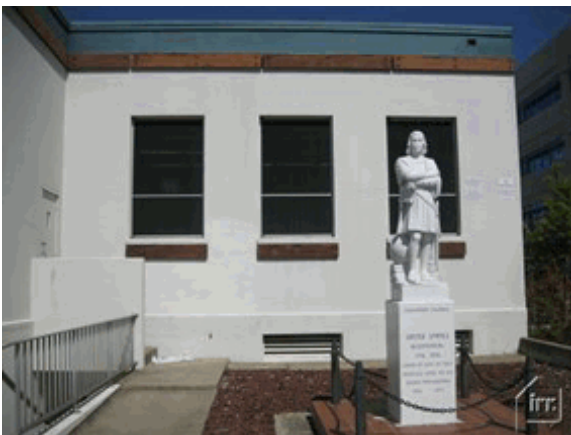
Eastern corner of the building
