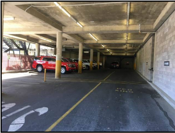
Basement parking garage
