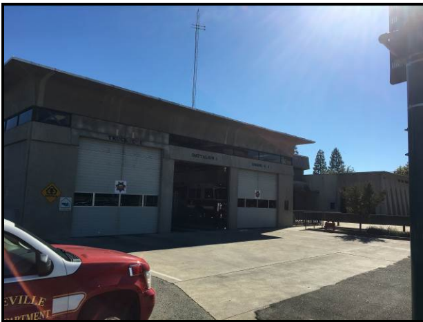
Fire engine bay
