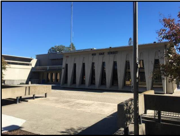
Northwest side of subject
