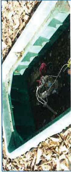
Valves placed centered in valve box, aligned square within the box, tagged and filled with drain rock.
