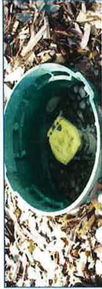
Quick coupler valves set 2-1/2" above finish grade in planting areas, placed centered within the valve box and anchored with an angle iron, 36" long.
