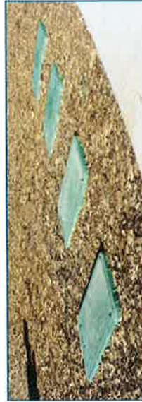
Valve boxes aligned and square with hardscape. Boxes are set at 2-1/2" above finish grade in planting areas and 1-1/2" above finish grade in turf areas.
