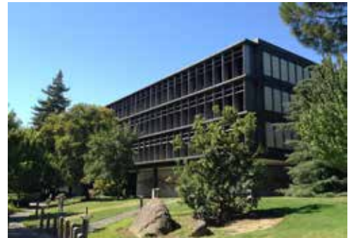
SMUD Headquarters Rehabilitation, Sacramento
