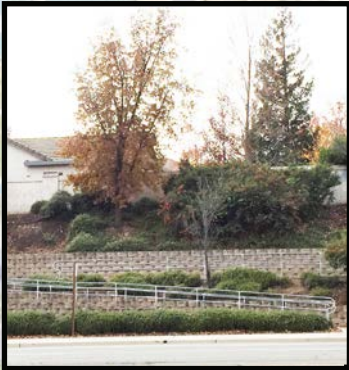
Slope groundcover planting
