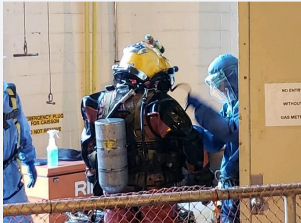
Photo c/o Charleston Water: Divers preparing to go 90 feet into raw sewage to search in complete darkness with their hands to find and identify obstruction
