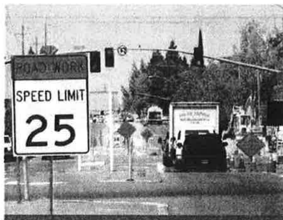
HDR performed CM on the City of Roseville's Cirby Way/ Riverside Road/I-80 Ramp Improvement Project
