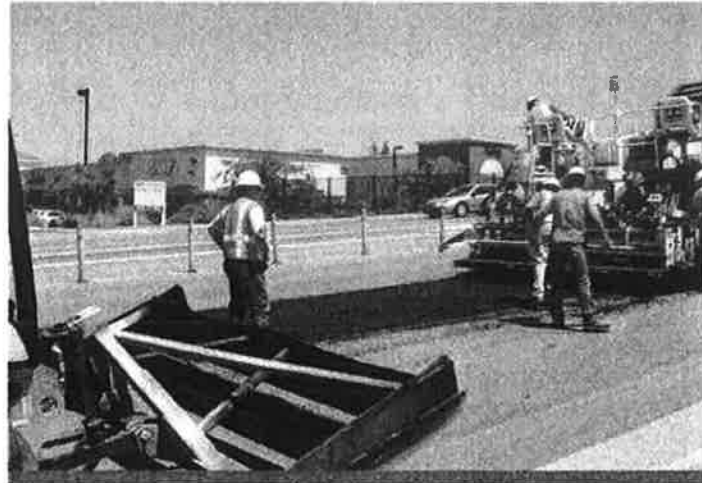
Construction crew at Cirby Way / Riverside Road / I-80 Ramp Improvement project site
