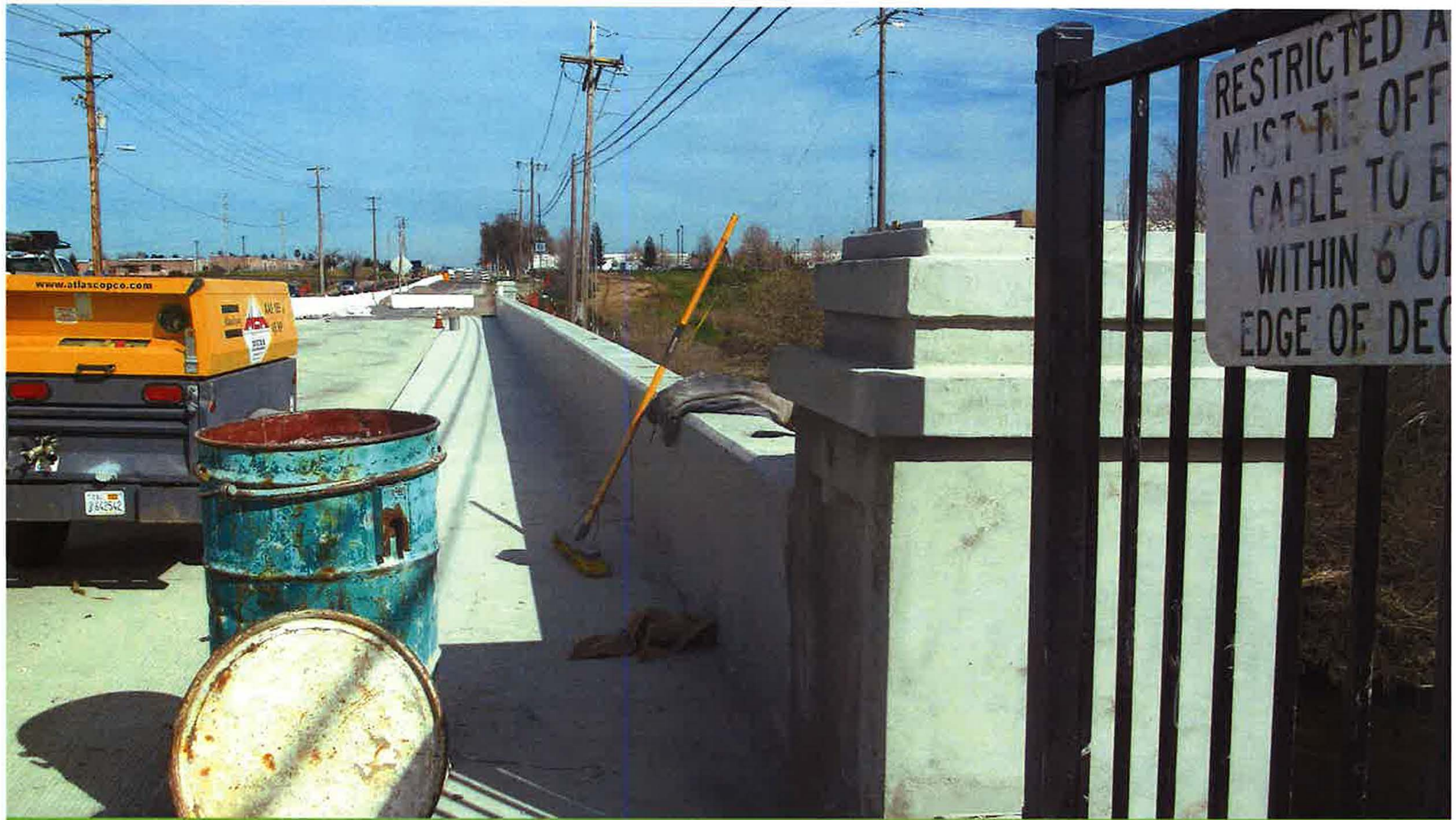
Industrial Bridge Replacement - After
