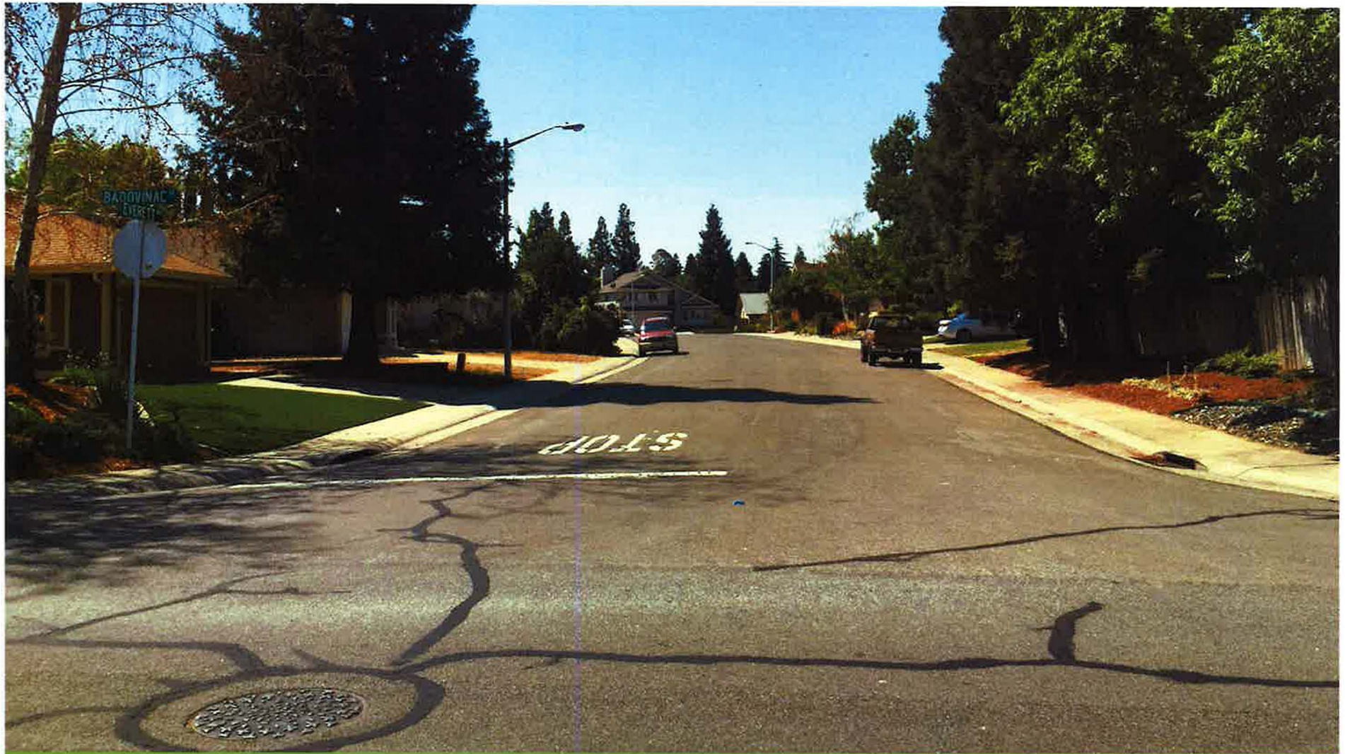
Residential Resurfacing 2016 - Before
