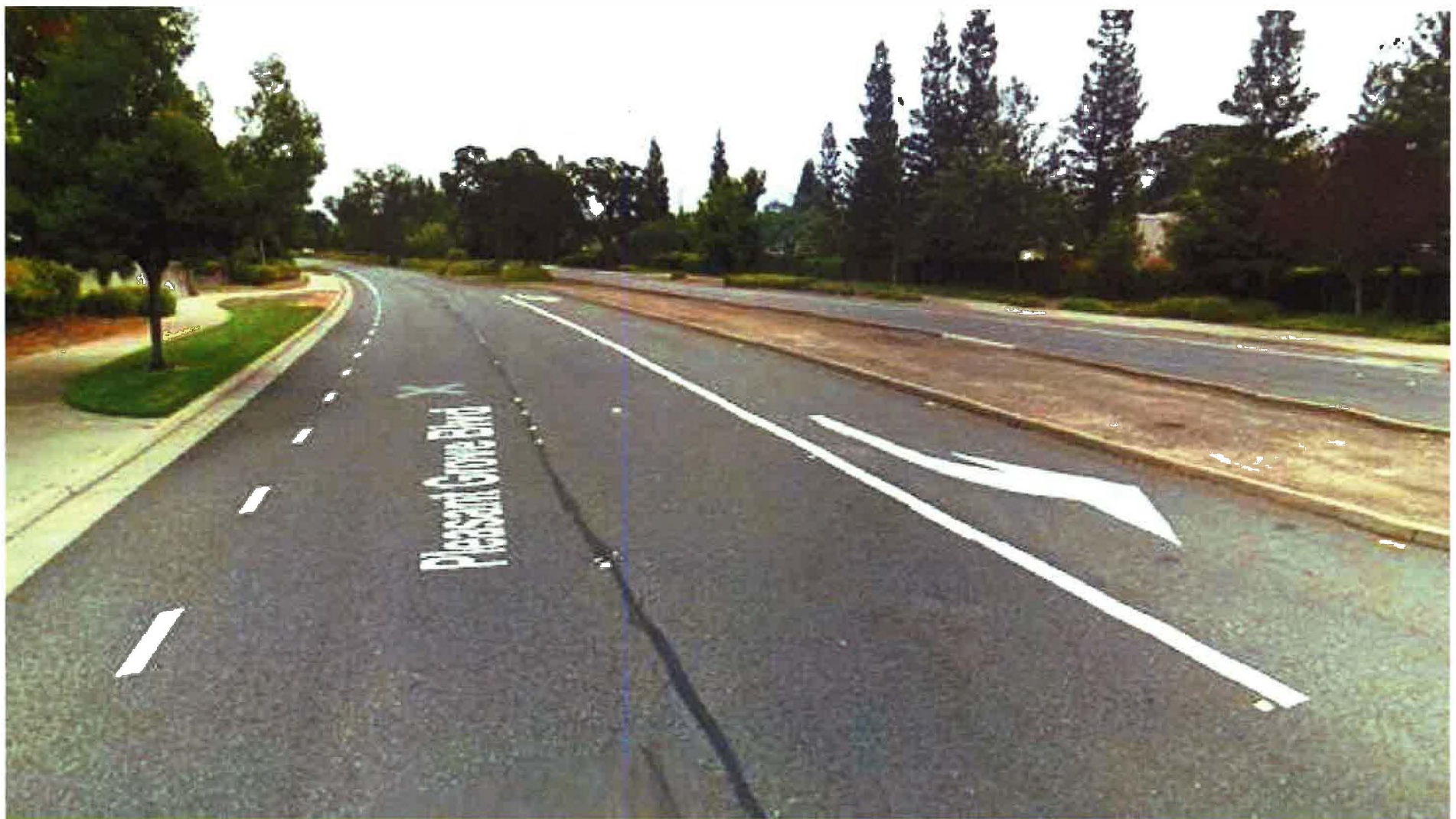
Arterial Resurfacing 2016 - Before
