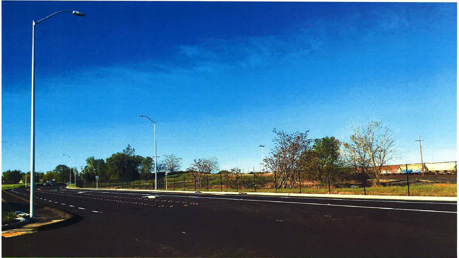
Roseville Road “S” Curve Realignment - After
