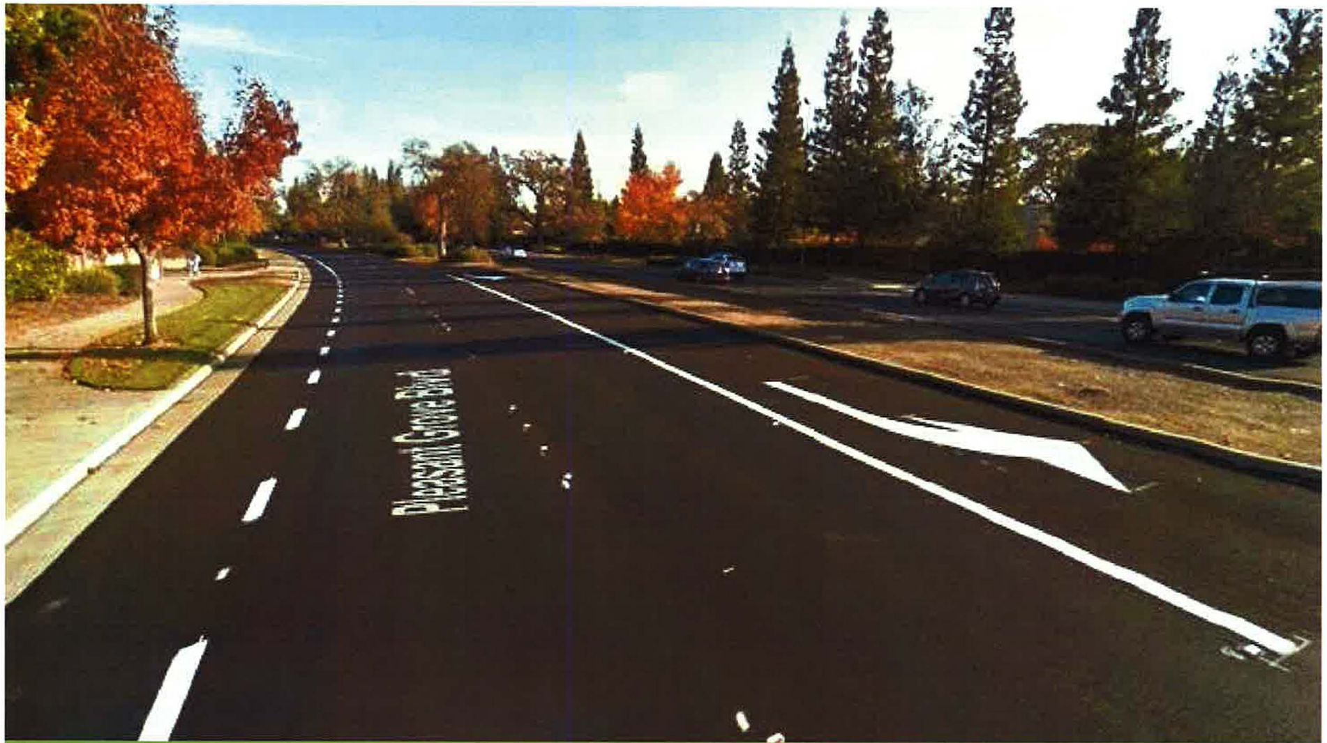
Arterial Resurfacing 2016 - After
