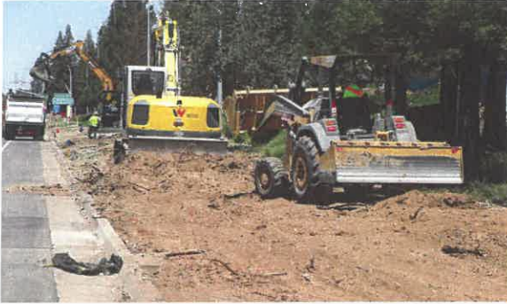
Clearing and Grubbing in Advance of Widening Work at Washington Boulevard
