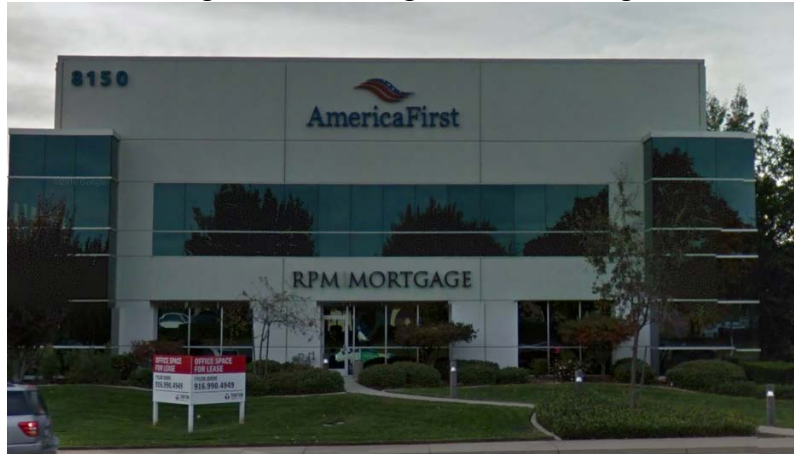
Figure 3: Existing Office Building
