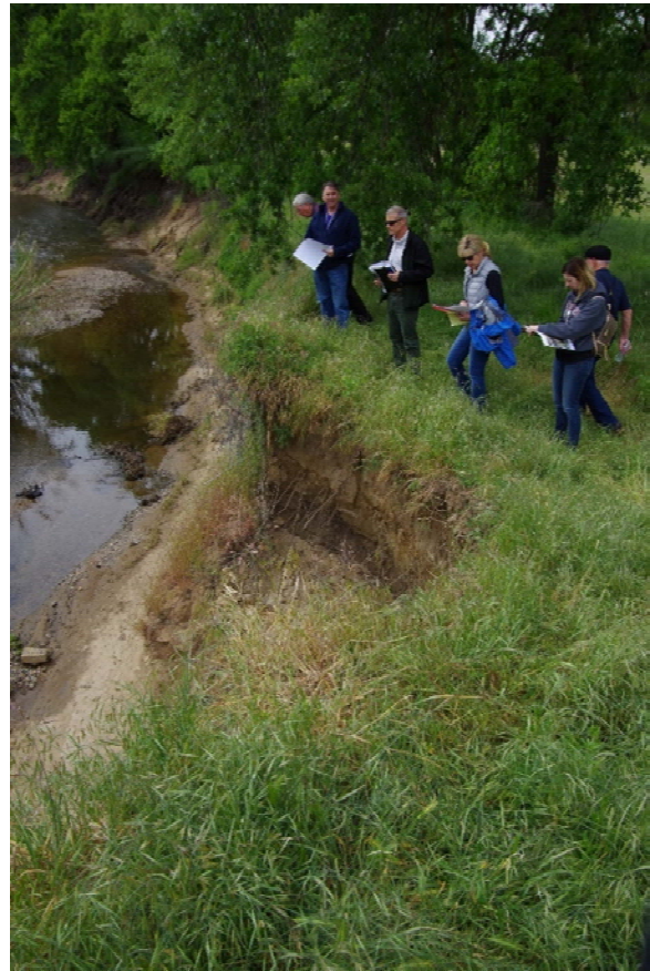
Photo 4-1: Site walk with property owner.
