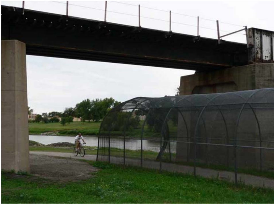
Figure 12: Integrated chain-link cover and fencing protects trail users along East Grand Forks National Recreation Trail in Minnesota; photo courtesy Stuart Macdonald
