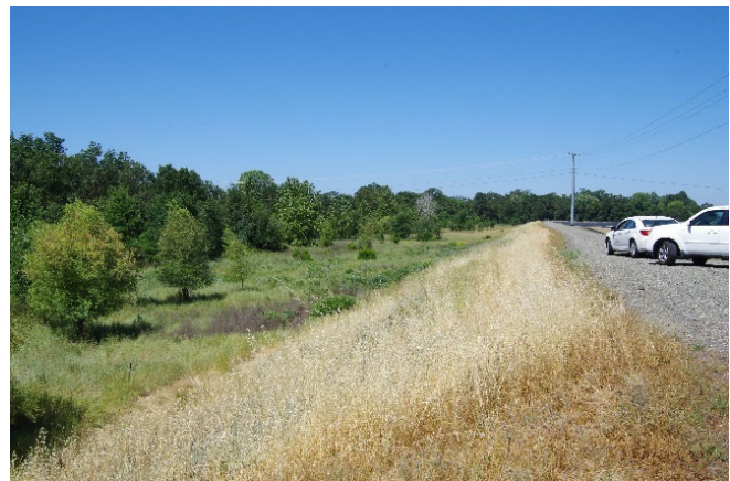
Photo 4-4: New levee at Roseville WWTP, looking west.
