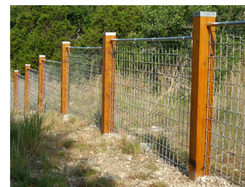
4' Hog wire and wood fencing
