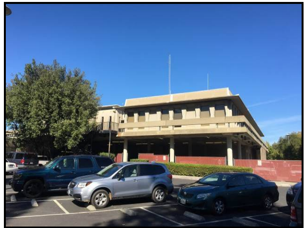
Southwest side of the building
