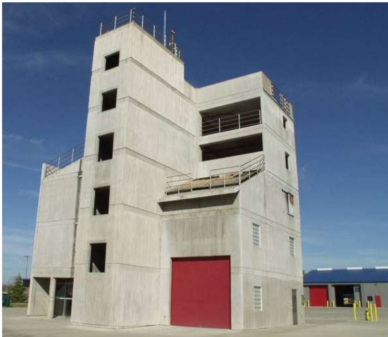
Figure 13-5. City of Roseville Fire Training Center
