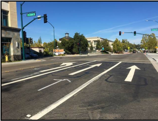
Looking north along Oak Street
