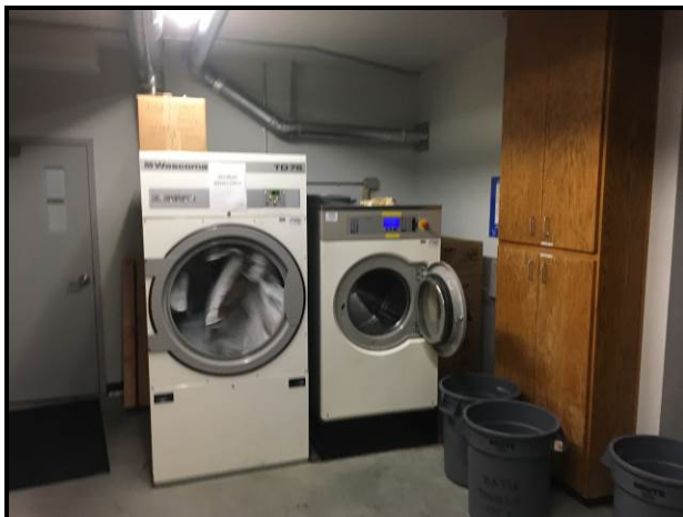
1 st floor laundry room
