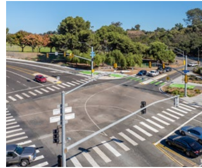
High-Visibility Crosswalk in San Diego, CA.
