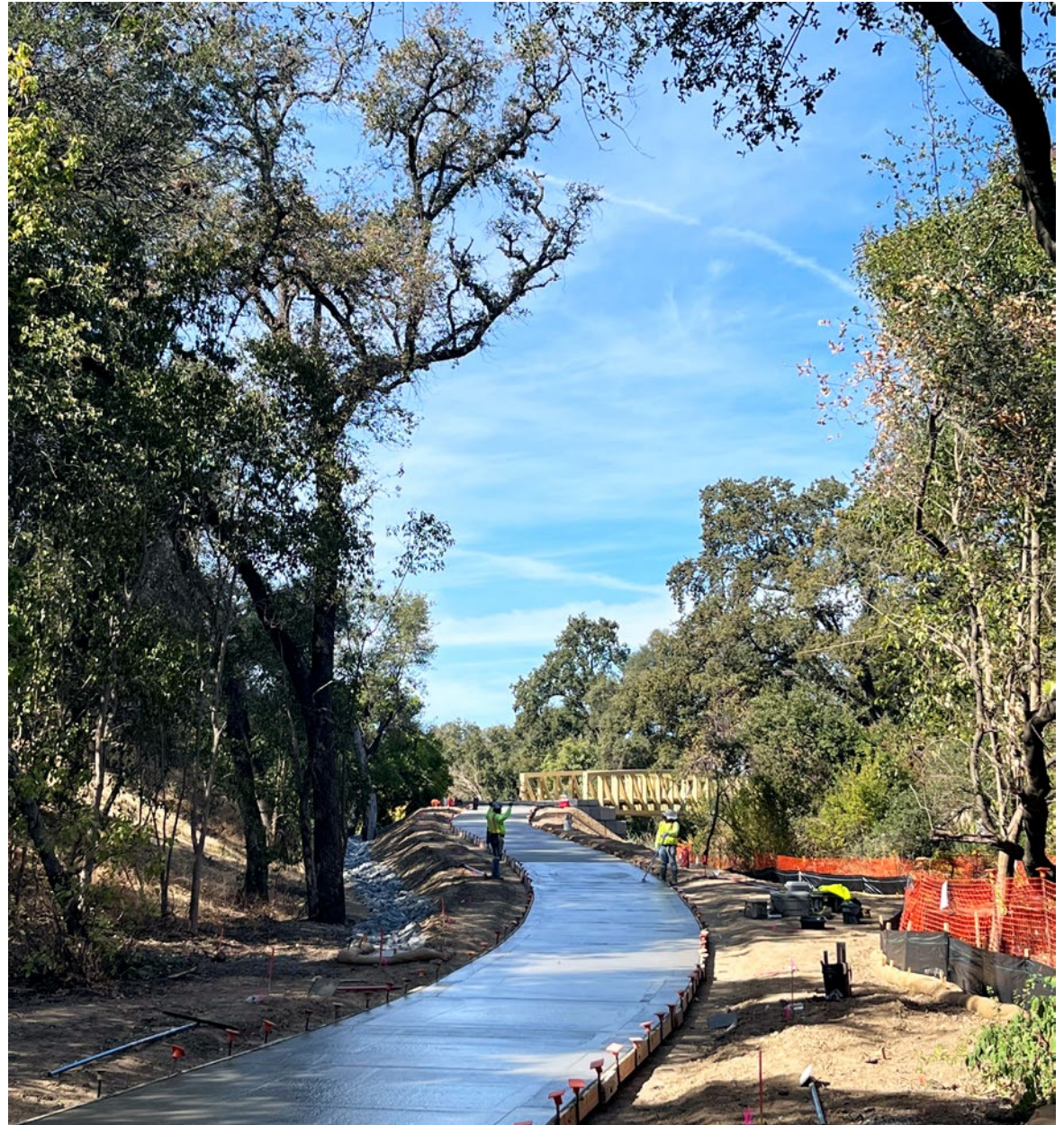
Dry Creek Greenway drainage and construction.
