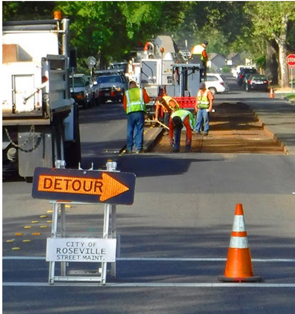
Street Maintenance crew reconstructing a section of Oak Street in Roseville.
