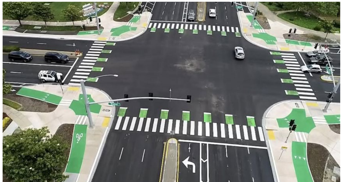
Protected Intersection in Fremont, CA.
