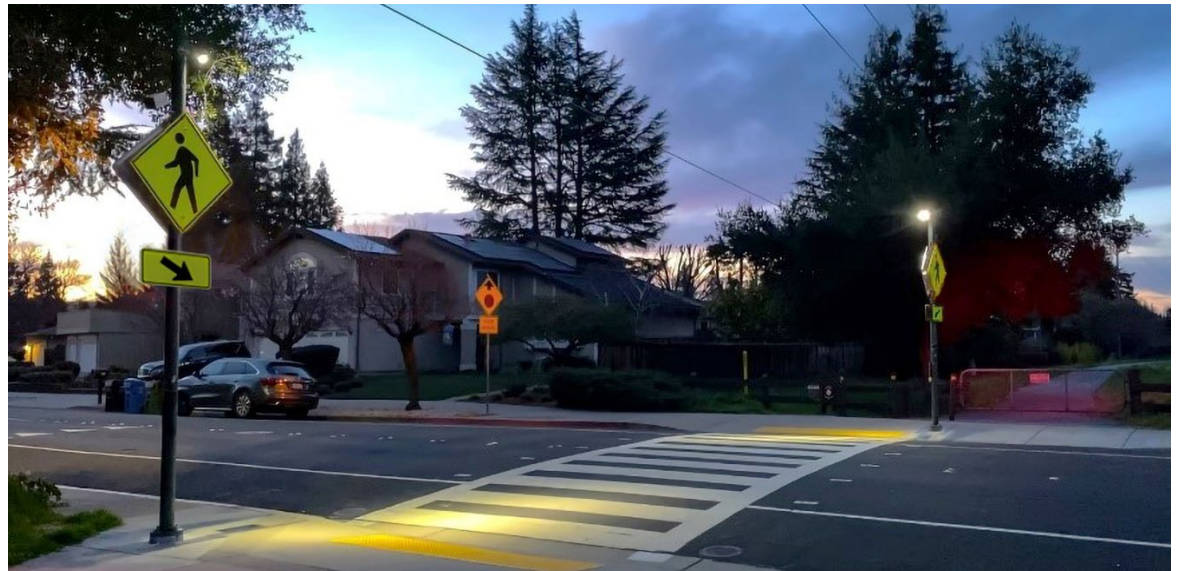
High-visibility crosswalk and lighting on Iron Horse Trail crossing in Danville, CA.
