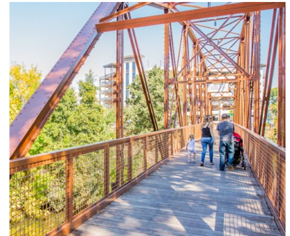
Grade-separated crossing in Roseville.
