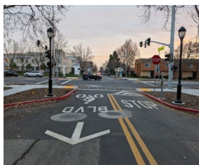
Intersection Daylighting in Richmond, CA.
