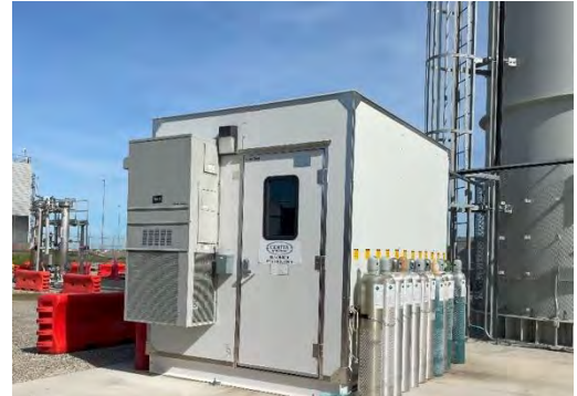
Figure 3: Cemtek CEMS at RPEAK
