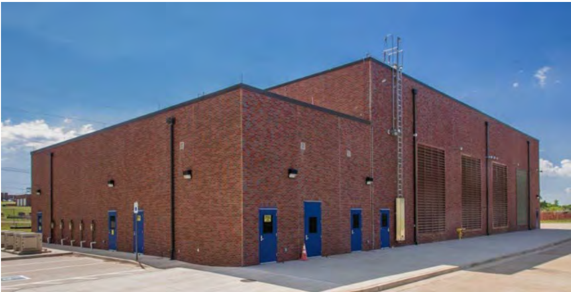
Tier 4 standby generators installed at the Draper WTP in Oklahoma City required a ceiling height of 35 feet and a full room working platform for O&M access of the emission treatment equipment.
