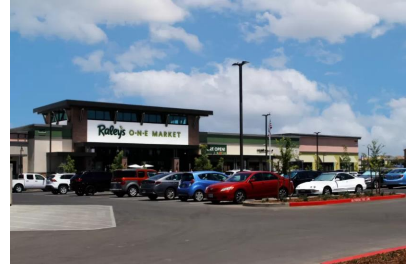
Plaza at Blue Oaks – Rayleys (recently constructed) 5351 Fiddymment Road
