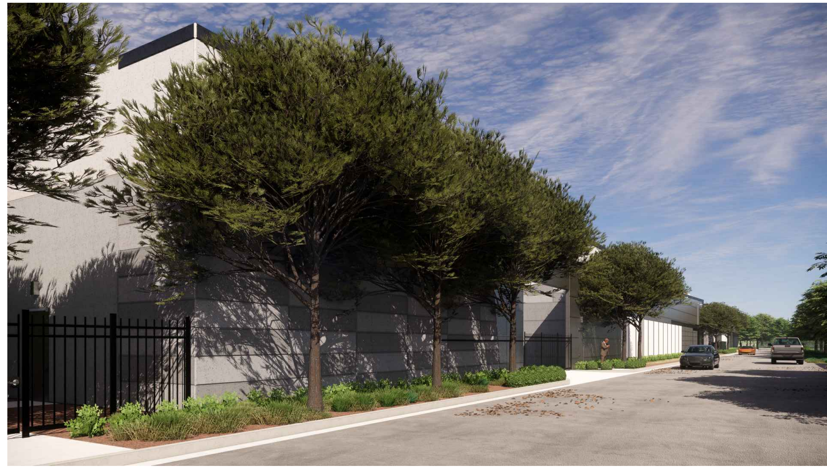
B: VIEW OF SOUTHWEST BUILDING CORNER
