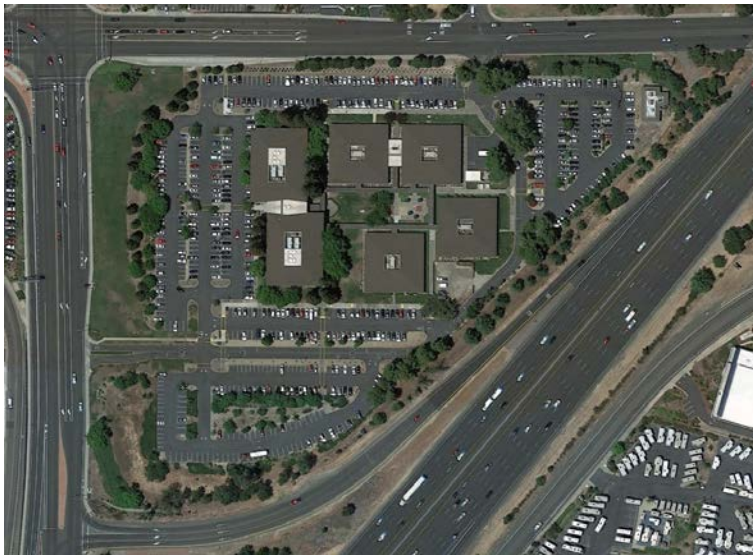
Figure 1. Project Location. The existing Kaiser Medical Office Building is located at the Southeast corner of Riverside Avenue and Cirby Way in Roseville, CA. Image credit: Google Earth
