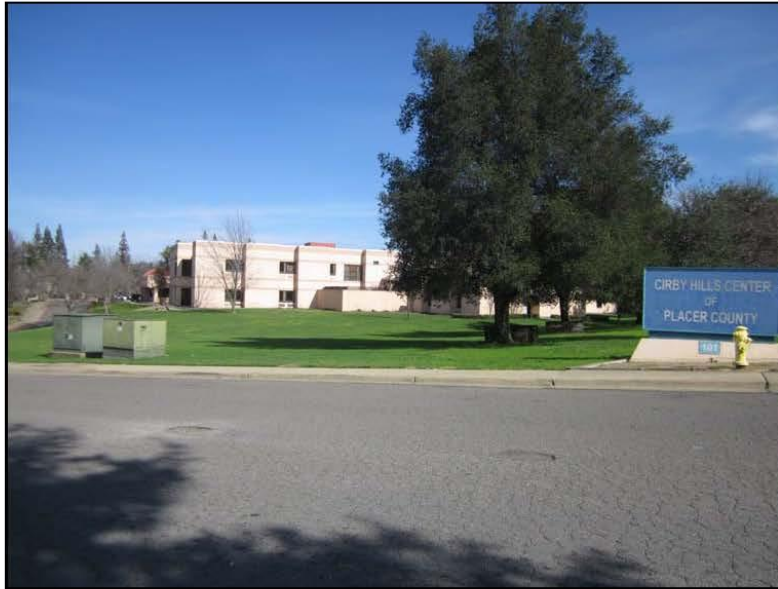
FIGURE 4.4-4 View of Telecare Corporation Health Care Facility along Cirby Hills Drive
