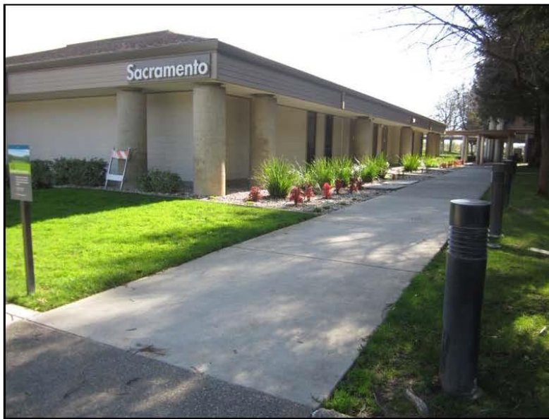
FIGURE 4.4-5 View of Existing Kaiser "Sacramento" Building
