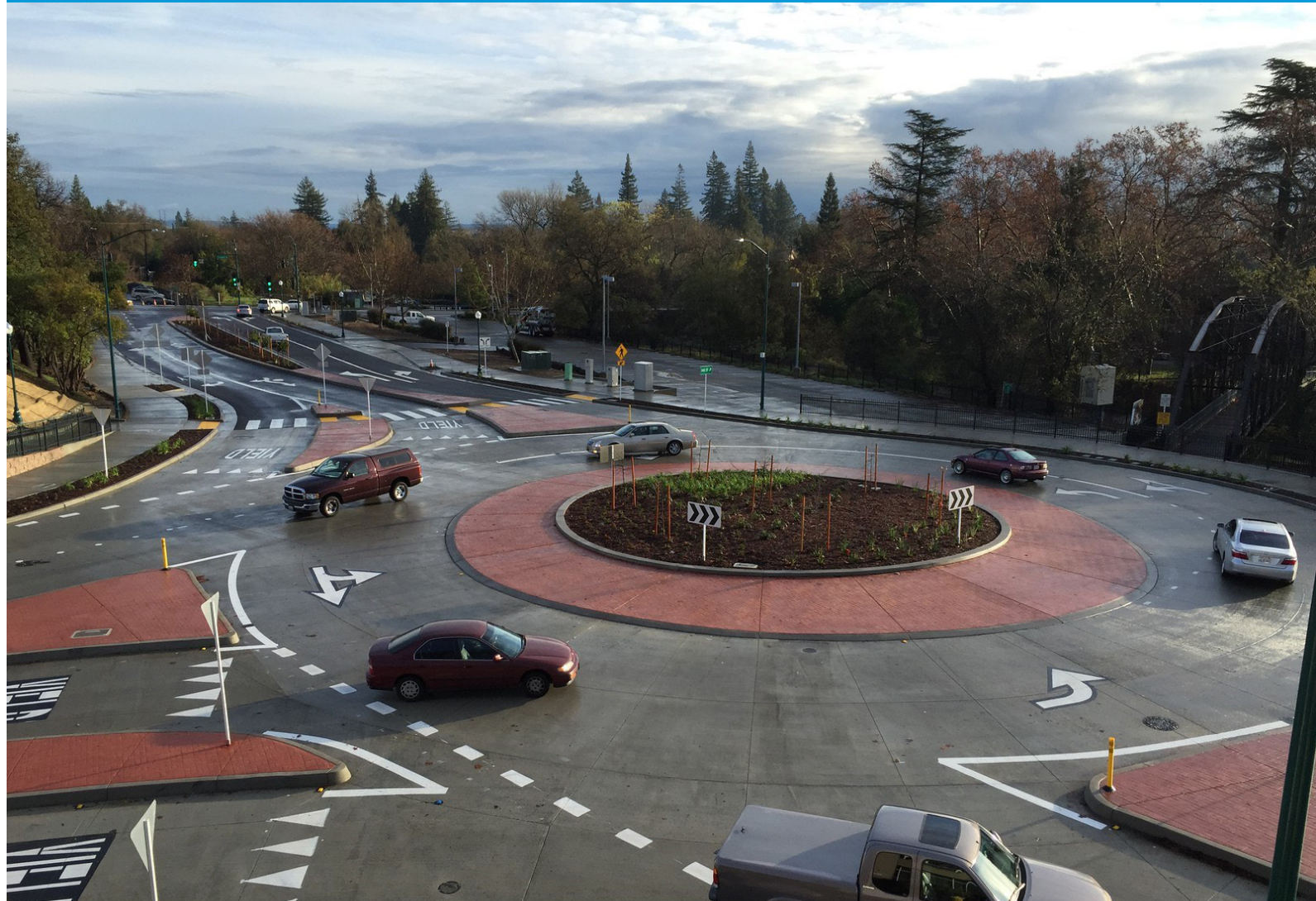
Downtown Roundabout, Roseville, California
