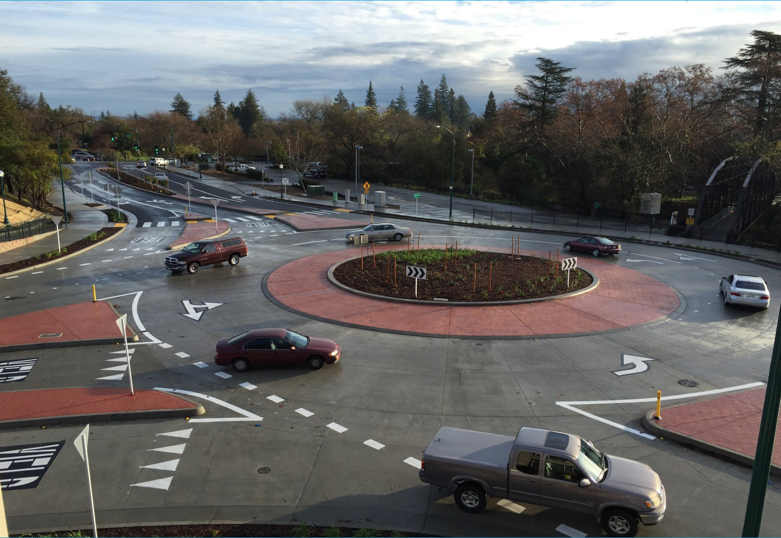
Downtown Roundabout, Roseville, California
