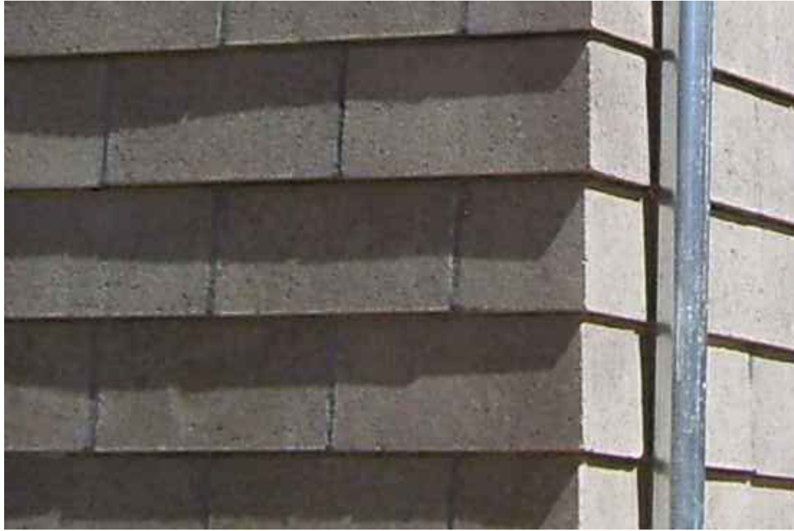
TRASH ENCLOSURE WALLS CONCRETE MASONRY UNITS, SHIPLAP PROFILE (SHOWN ABOVE, SEE BELOW FOR COLORS) BODY COLOR: MATCH OTHER PRECAST (EARTHTONE BROWN/LIGHT BEIGE, BASALTITE STD. 113 OR SIMILAR) CAP COLOR: STD. WALL CAP, DARK BROWN (BASALTITE STD. COLOR 408 OR SIMILAR) METAL DOORS: LOUVERED OR CORRUGATED (HORIZONTAL), SEE BELOW FOR PAINT COLOR.
