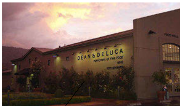
Vines & Wall Trellis Clerestory Windows Standing Seam Roofing
