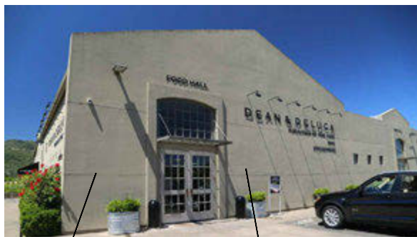
Imperfect Smooth Plaster Finish w/ Horizontal Reveals Peaked Element Counterpoint
