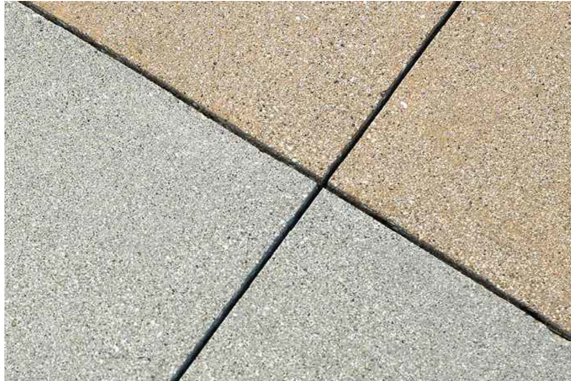
DECORATIVE CONCRETE ACID-ETCH FINISH (WEATHERS' NEW CONCRETE TO EXPOSE FINE AGGREGATES AND ELIMINATE SHEEN AND GLARE OF NEW PLAIN CONCRETE) SHOWN OVER PLAIN AND INTEGRALLY COLORED CONCRETE
