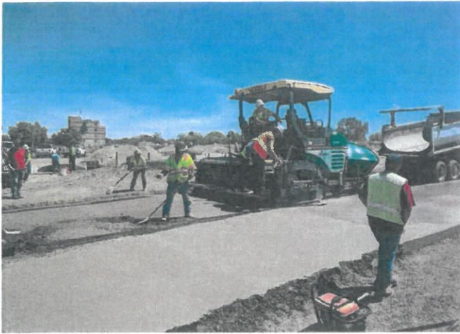
The City is receptive to innovative pavement techniques Roller Compacted Concrete Project - City of Roseville
