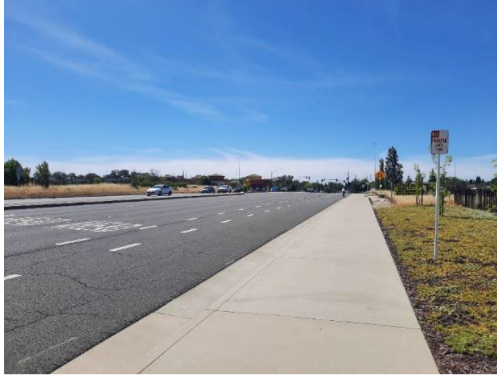
Figure 4.5-4. Overview: northern Project Area boundary at Foothills Boulevard (view southeast, June 9, 2022).
