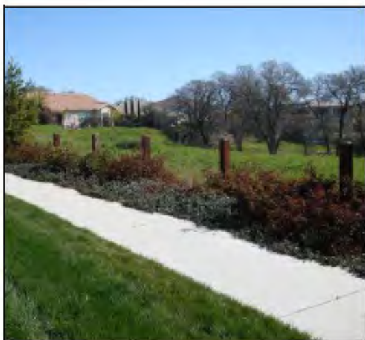
Post and cable fence
