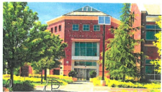
Top: State Capitol East Annex Fan Room Replacements Bottom: Placer County Finance Administration Building
