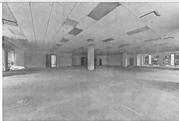
TYPICAL UNIT INTERIOR
